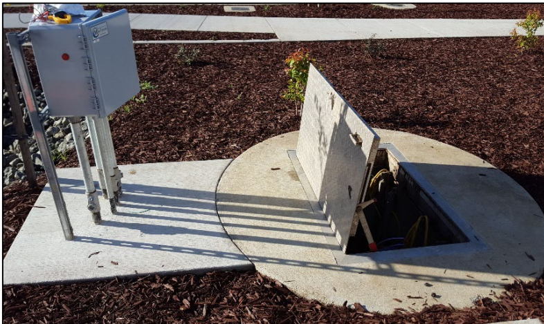
Jensen Pump Stations recommends that the panel is mounted as close to the wet well as possible to limit voltage loss in cables and provide convenience for continued maintenance.
