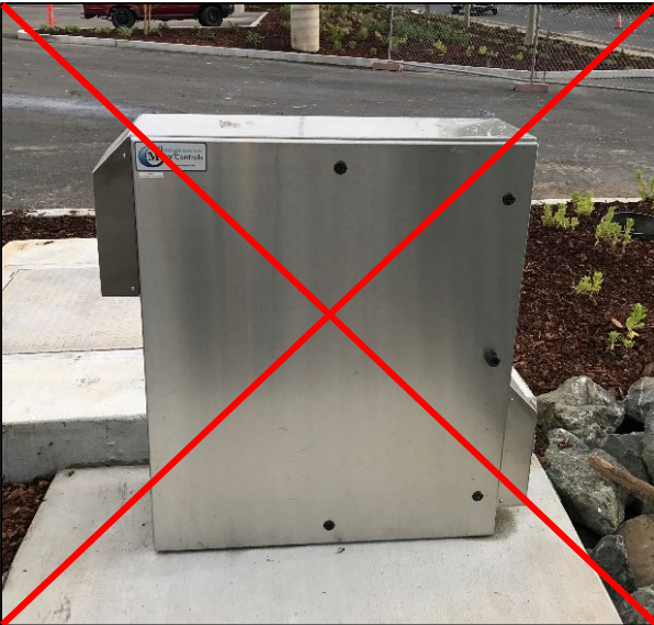
Do not install the enclosure directly on the ground or a concrete slab! Moisture and debris will damage the internal components.
