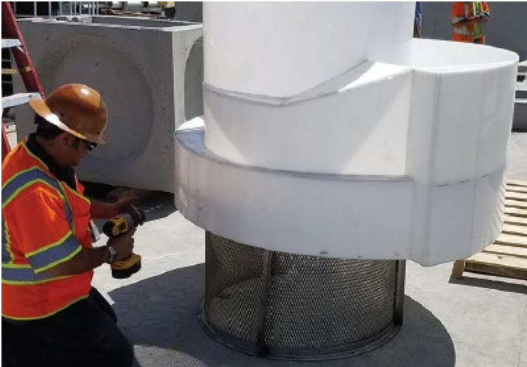
Figure 4. Assembly of screen cylinder and integral inlet and bypass & oil baffle, for insertion in a small 60-in ID Inline JDS unit
