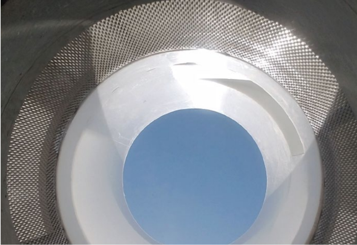
Figure 2. Bottom Up View of Separation chamber, Expanded screen cylinder and HDPE Inlet riser – Inline Unit
